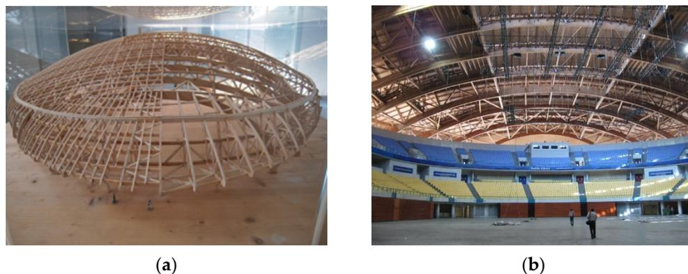
**Figure 9.** Example of timber structure in Portugal: (a) Altice Arena (Utopia) structural scale model; (b) Altice Arena, inner view.
