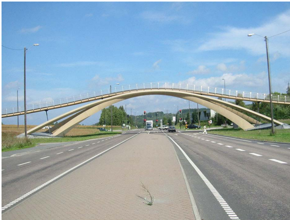
[Large curved beams]
